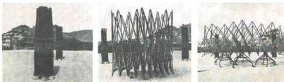
Fig. No. 104 Expandable truss technique developed by Emilio Pinero of Madrid. Segments packaged as compact bundles. Unfolded in wheeled trolleys and joined together to provide dome structures up to 300 feet in diameter.
