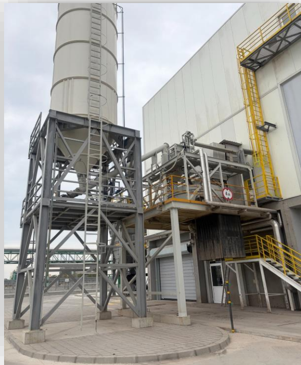
Silos cementa i mikser
